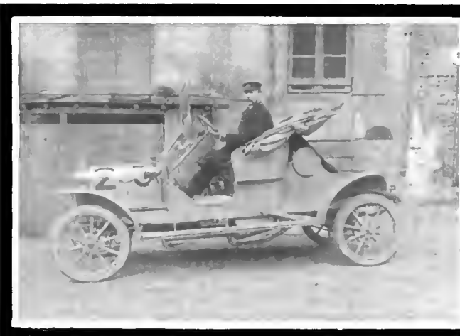
Turicum Four-Cylinder with Single Chain Drive
